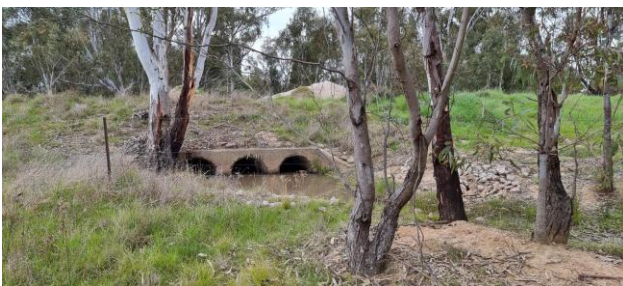
Figure 5. Culverts under Burma Crt
