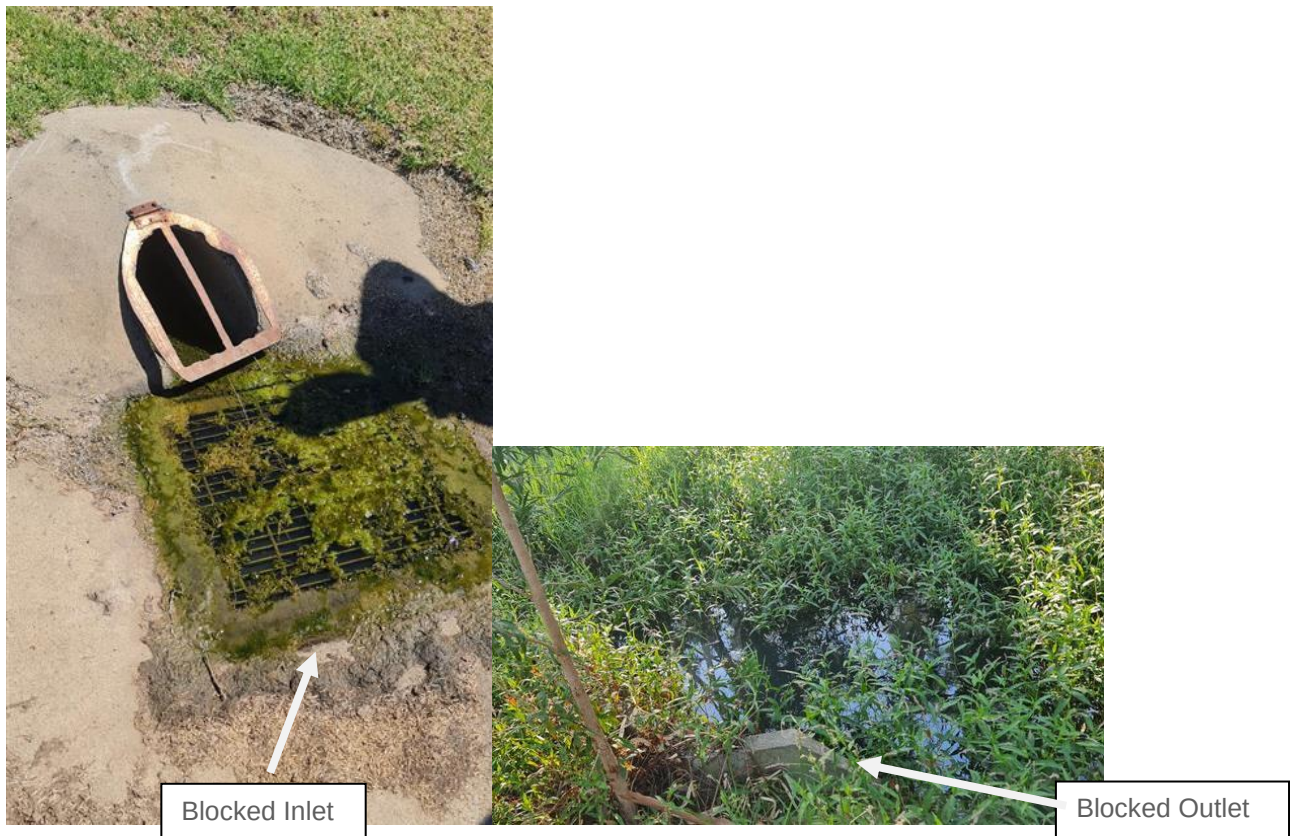
Figure 14. Outlet Pipe Inlet and Outlet (February 21 st 2025)
